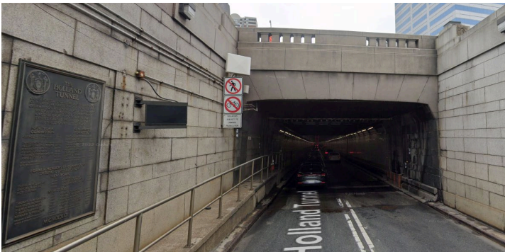
Figure 5 Entrance to Holland tunnel, Jersey City NJ
